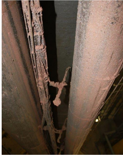
Annex C Fig. 3: Oxide formation next to the DHR-system
