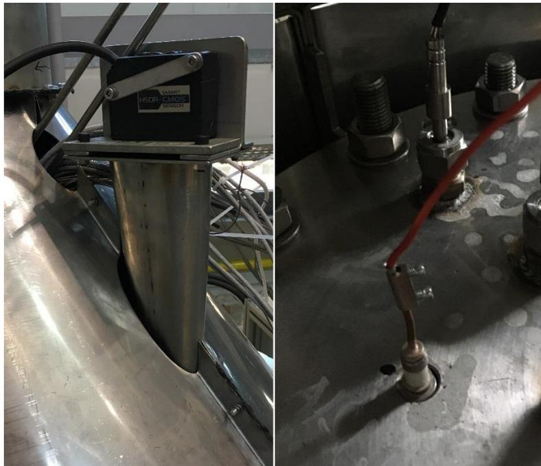
**Figure 3-6: Lead level sensors; laser level measurement (left), contact level sensor (right)**
